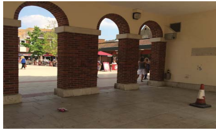
Existing open undercroft of Old Town Hall today
