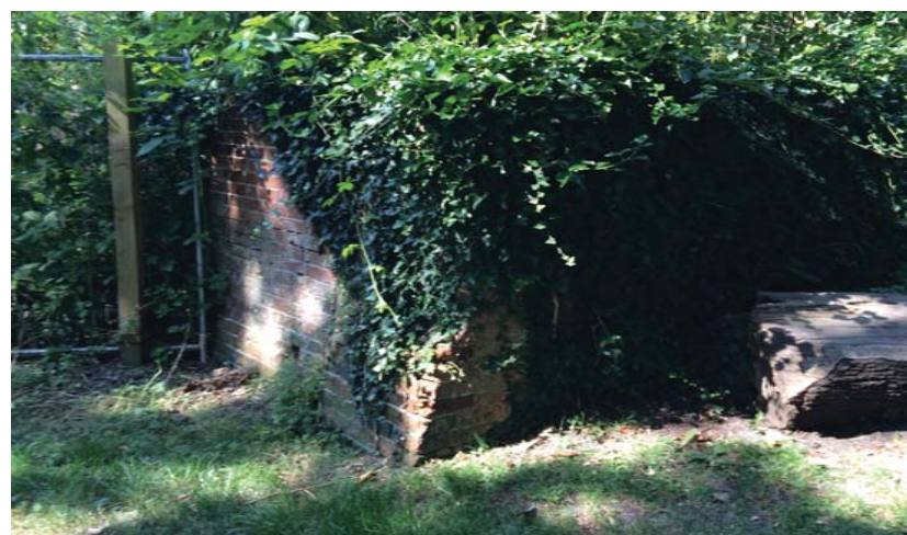
Existing overgrown land burying the scheduled monument at the Druiitt Gardens/Bank Close boundary
