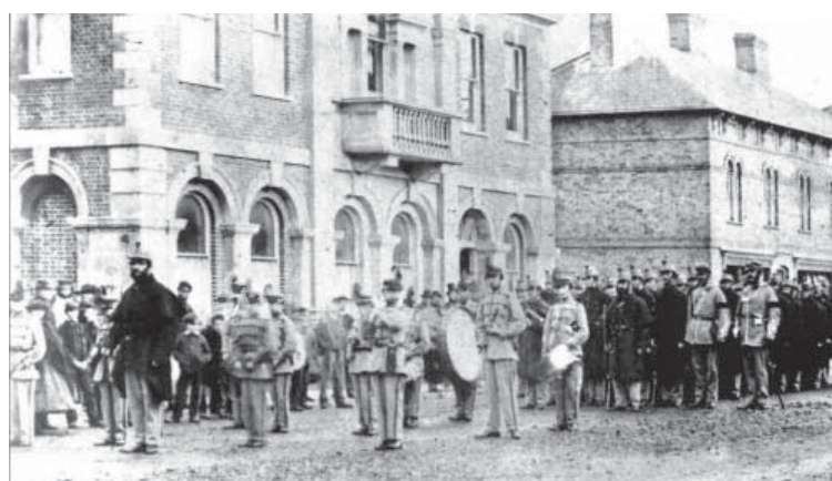
1860 image showing previous infill of ground floor
