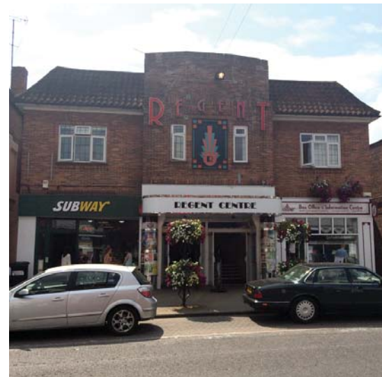
Existing Regent Centre Shopfront
