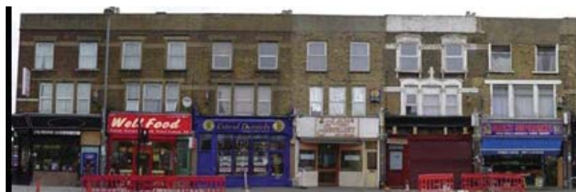
High Road example before frontage enhancements
