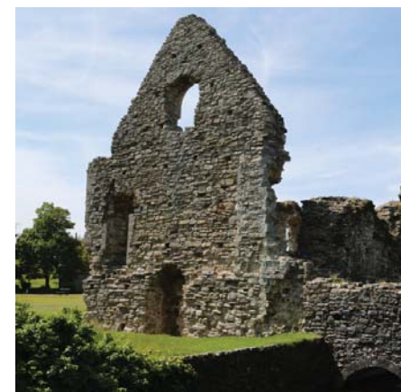
The Constable's House
